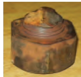
Damaged shrink fit bolt after removal
